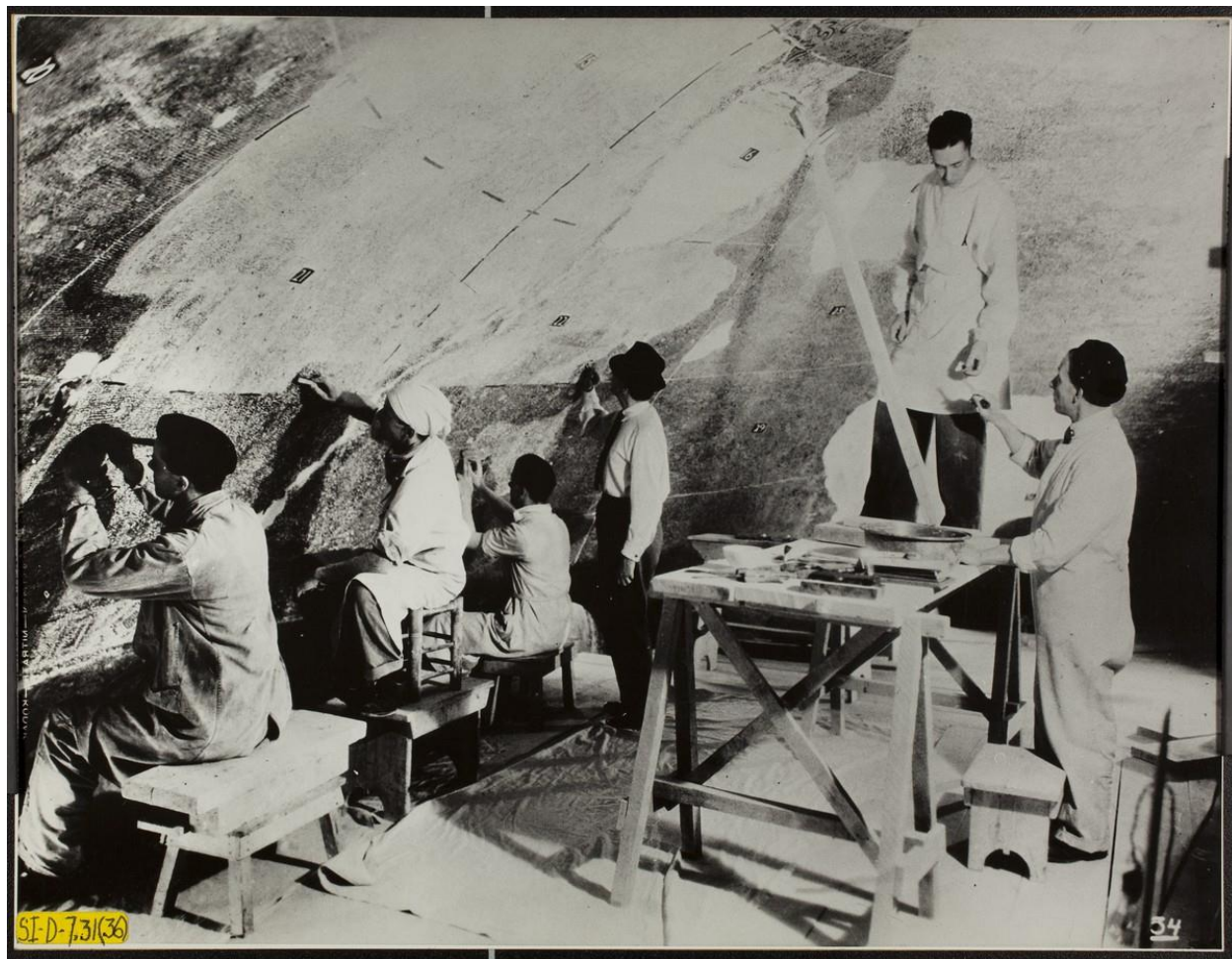
Fig. 4. Apse, group at work on scaffold, 10 July 1936. (Source: Dumbarton Oaks)
